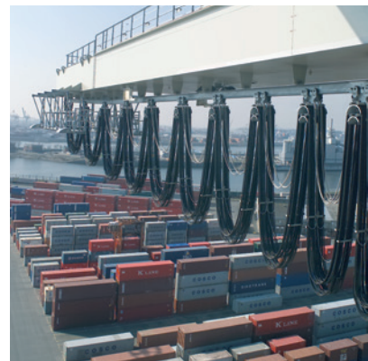
Supply of the crab on a fast travelling STS-container crane
